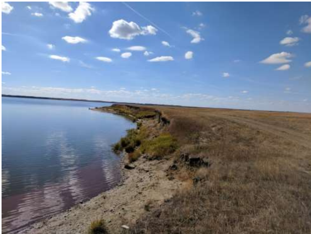
PHOTOGRAPH NO. 13147-02 Surficial slumping and erosion along shoreline. Approximately at west end of Phase I
